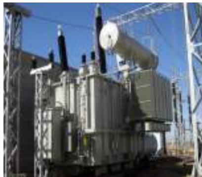
Gambar2. 8 Transformator Daya
