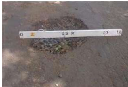
Gambar 2. 31 Lubang (Pothole)
