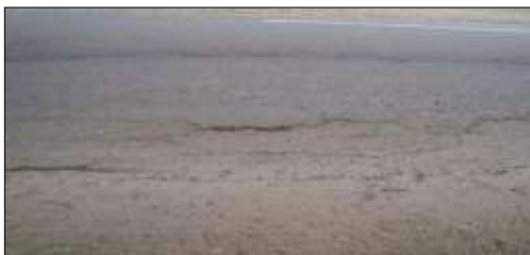
Gambar 2. 13 Cekungan (Bumb and Sags)
