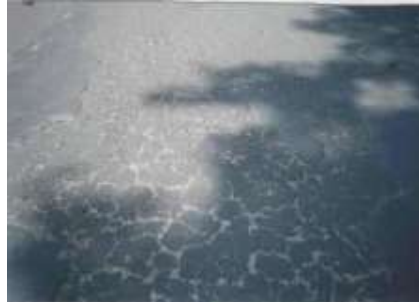
Gambar 2. 43 Pelepasan Butir ( Weathering/Raveling )
