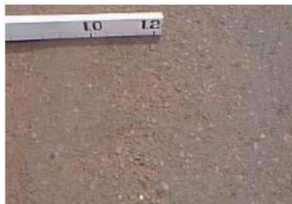
Gambar 2. 29 Pengausan Agregat (Polised Agregat)
