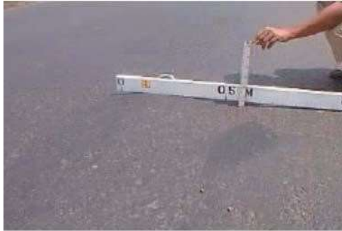
Gambar 2. 35 Alur ( Rutting )
