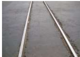
Gambar 2. 33 Rusak Perpotongan Rel ( Railroad Crossing )
